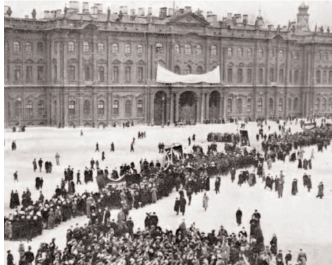
Demonstration at the Winter Palace
